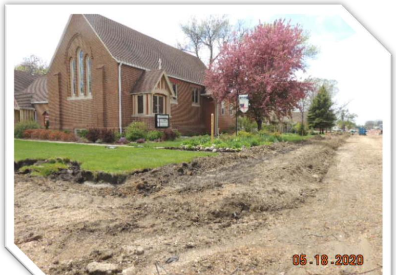
Sixth Street construction has removed the sidewalk, but spared our pollinator garden so far.
